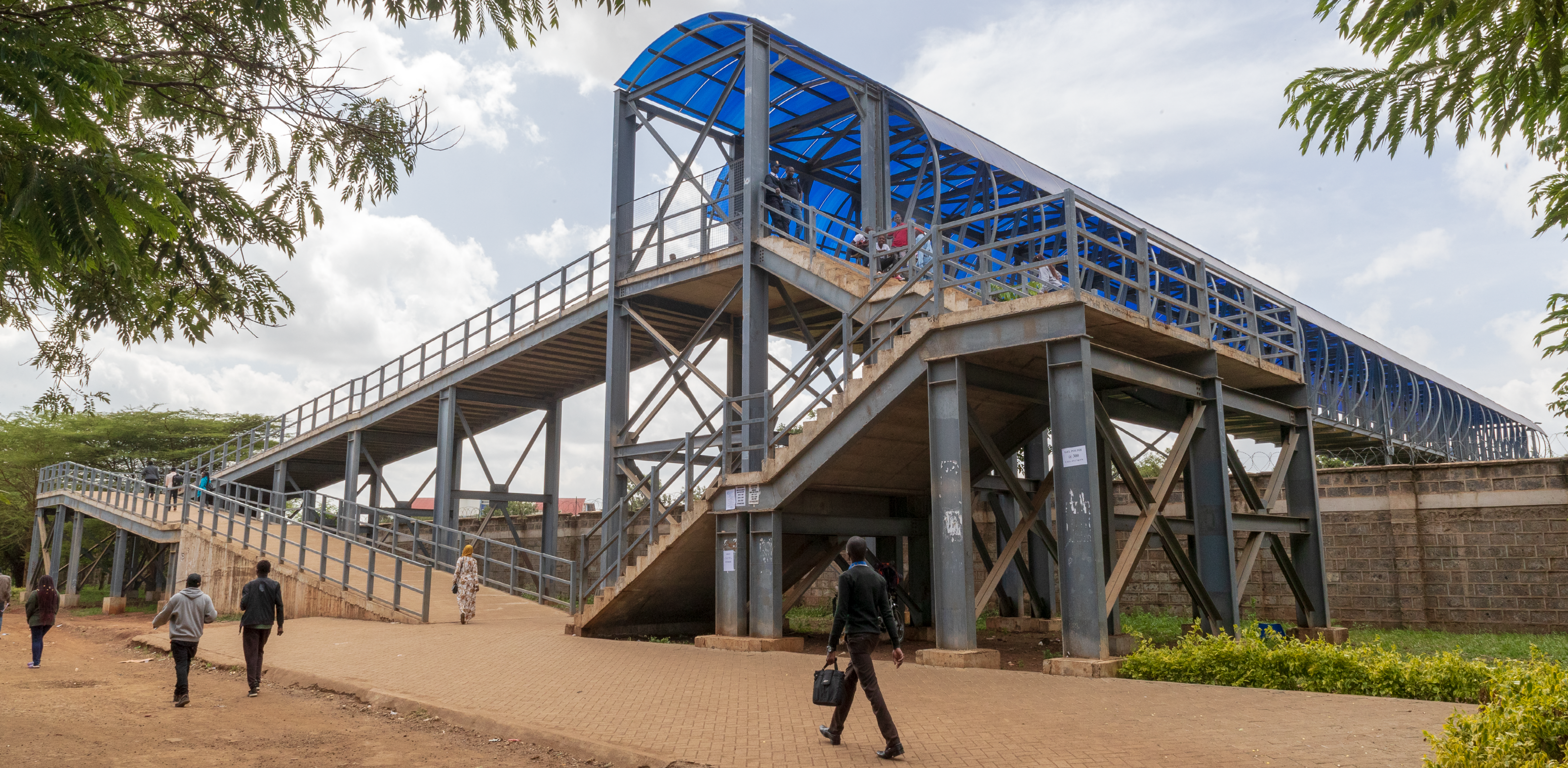
Kenyatta University, Nyayo Railway-Cross foot bridge
